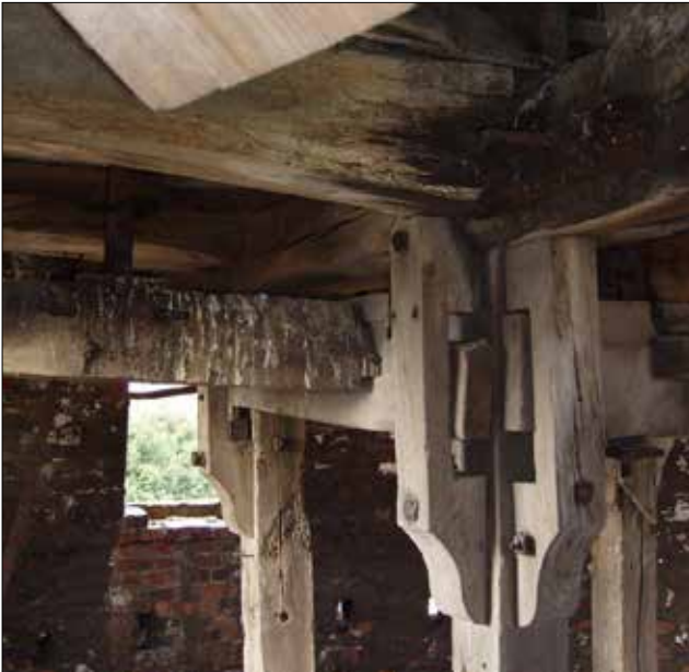
A view of the finely-made timberwork on the 3rd floor in 1989, showing elm uprights supporting the heavy framework which carries the millstones and enables them to be adjusted.
