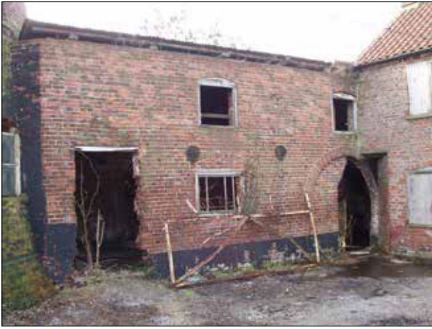
The listed ancillary mill building at Hewsons Mill in 2009. Note the partly-blocked waggon opening on the right
