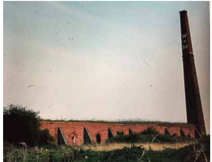
Fig. 7 The Hoffman-type kiln which survives at East Halton – looking east (Geoff Bryant)
