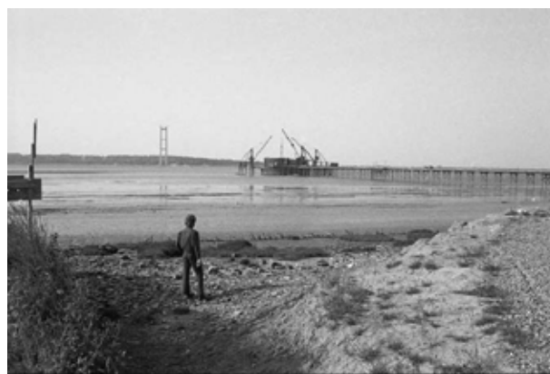
The caisson used to construct the southern tower
