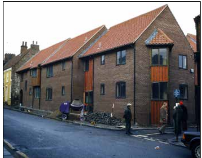
New residences on the High Street - St.Peter's Court, January 1981 (photo John: French)
