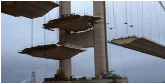
Sections of roadway being lifted into position
